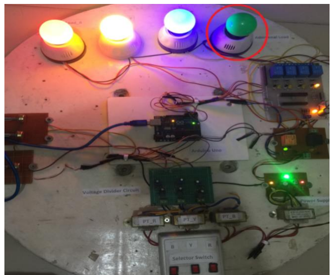
Fig. 16. (b) Turning off the bulb on the right side indicates that the additional load has been disconnected from the Red phase.
